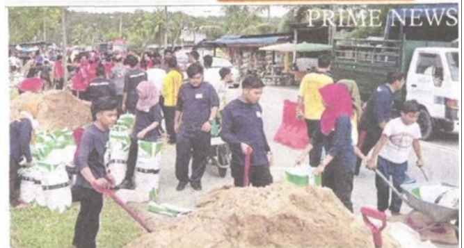
Armed forces personnel helping to build sand embankments in Kampung Panchor, Taiping, yesterday. Pic courtesy of Civil Defence Department.
